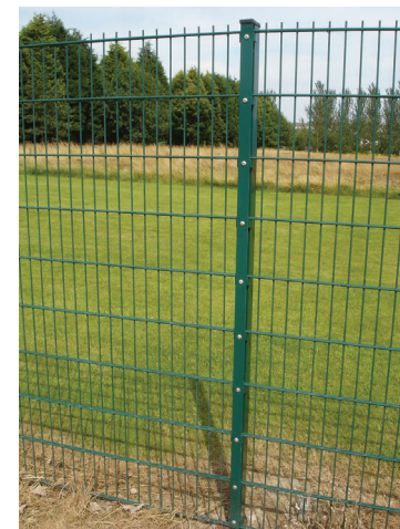
Image of east boundary fence at student blocks.
